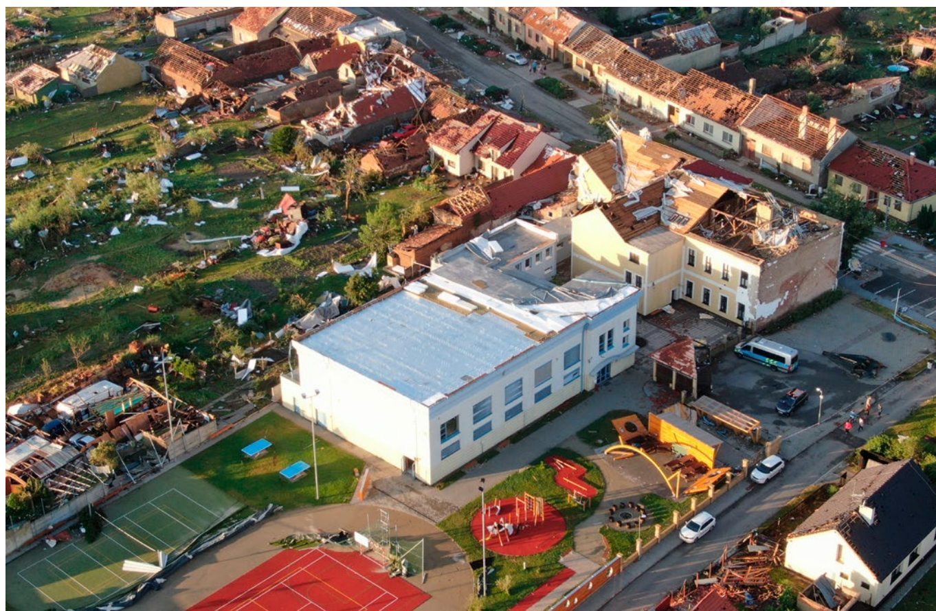
The state of the school building in Hrušky after the tornado in June 2021
